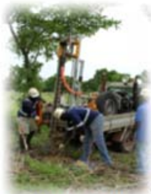
Auger drilling
